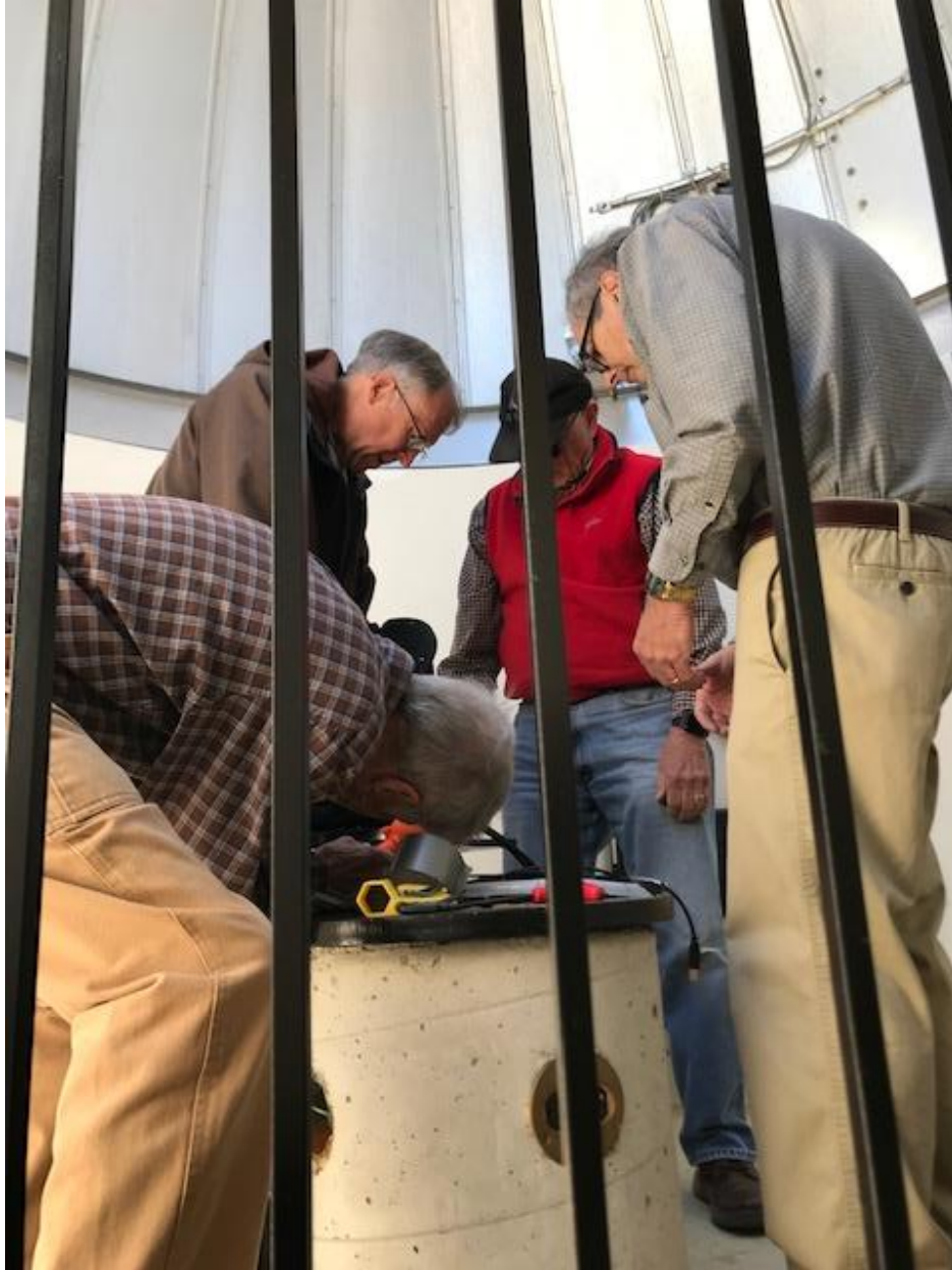
Figure 2. From L to R, Charlie Burke (bending), Brian Twohig, Gary Walker, and Hank Ricci work on the base of the PlaneWave telescope mount as part of installing the 16” spacer. The bars are not prison bars, but rather part of the railing leading up to the WSO dome. 😊
